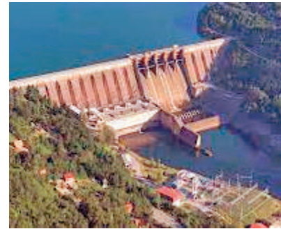
Bajina Bašta power station
