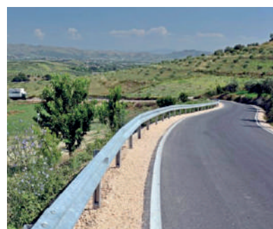
Recently upgrade rural road
