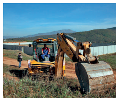
Work on the access road
