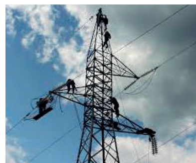
Transmission pylon installation
