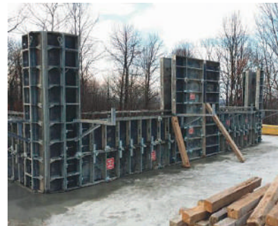
Building new pumping station
