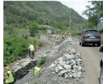
Upgrading a feeder road
