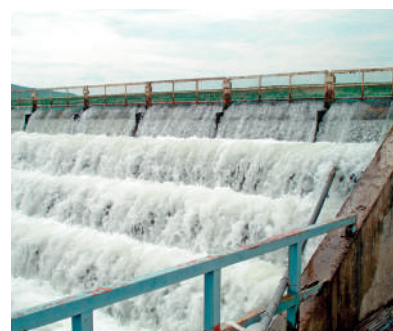
Iber canal, Pristina water source
