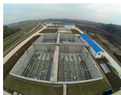
Bijeljina wastewater treatment plant implementation
