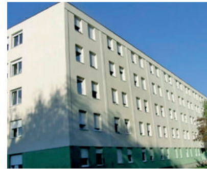
Refurbished student accommodation
