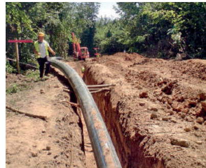
New pipe laying
