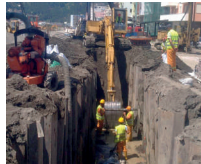
Laying new pipes in Shengjin
