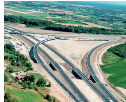
The interchange photographed just after construction completion
