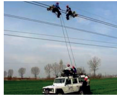
New overhead line installation
