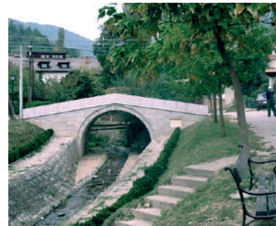
Vranje – open sewage channel
