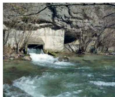
Untreated sewage discharge into River Lim in Berane
