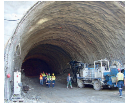
Construction of Vijenac tunnel
