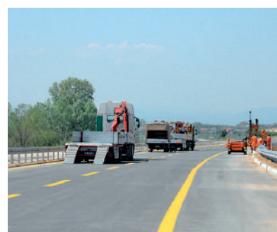
Construction is ongoing
