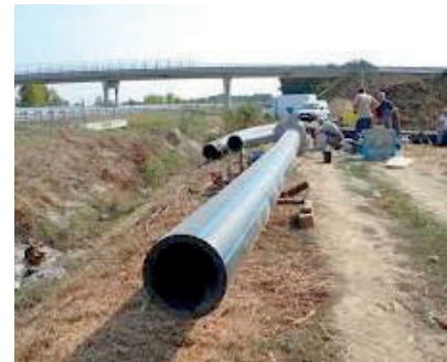
Pipe ready for installation
