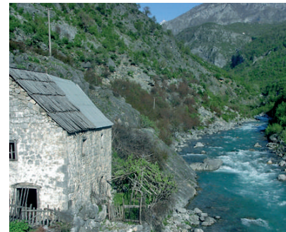
Rural water supply
