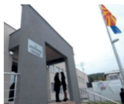
Kumanovo Prison construction completed
