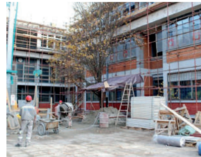
Thermal insulation to be fitted in school refurbishment
