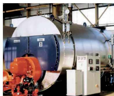
Greatly improved efficiency from a new boiler
