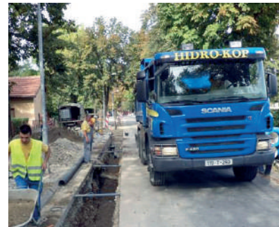
Laying new pipes in Banja Luka
