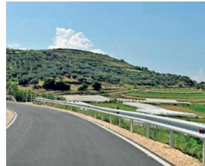
Upgraded road with new crash barrier
