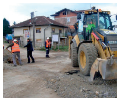
Work on new pipes
