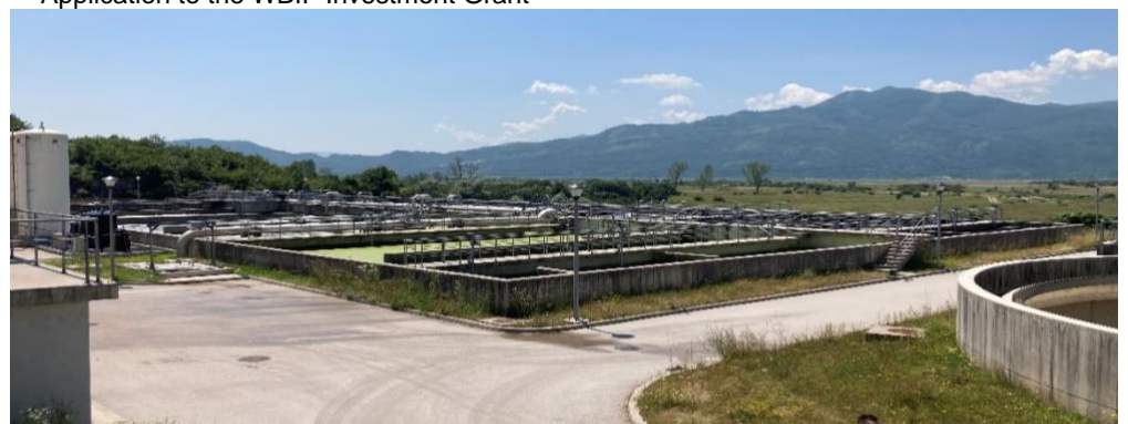
Nikšić wastewater treatment plant
