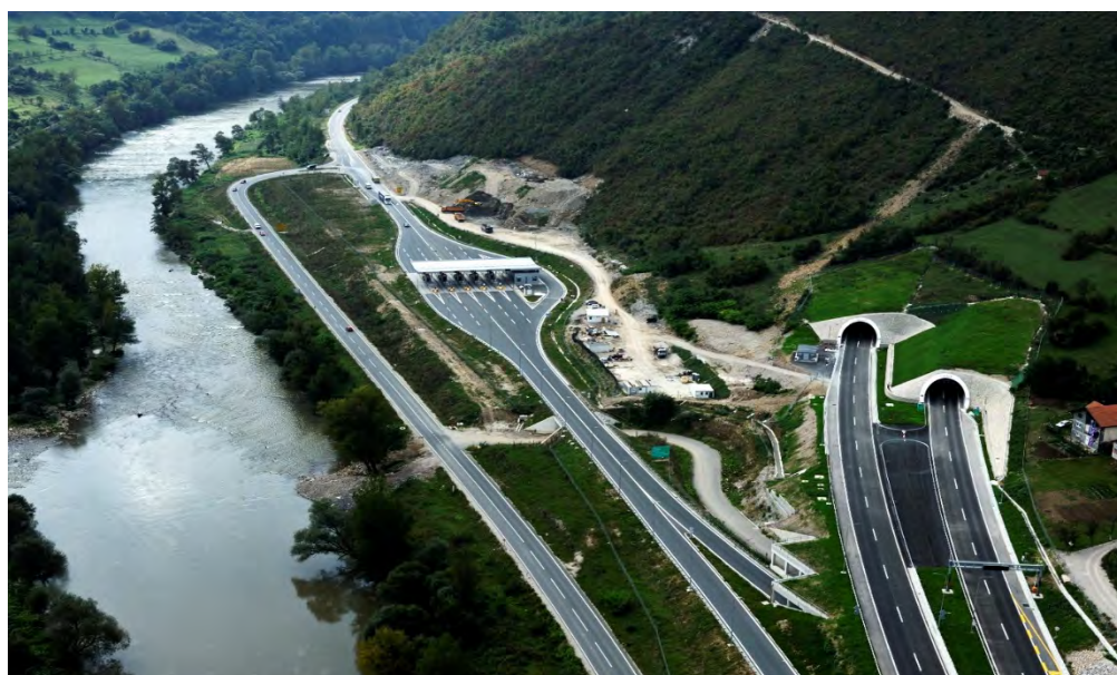
Completed motorway section on CVc in Bosnia and Herzegovina.
