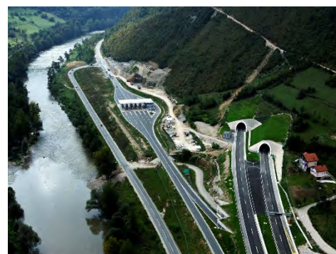
Corridor Vc in Bosnia and Herzegovina.
