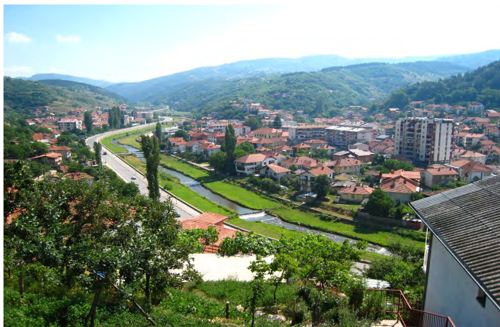
Existing road through Kriva Palanka, towards Deve Bair.
