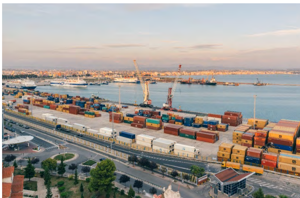
View of Durrës Port, container/logistics area.
