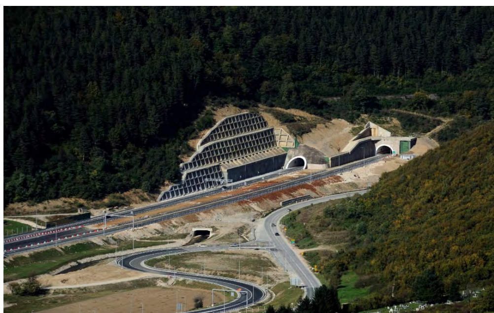
Completed motorway section, including tunnel on CVC in Bosnia and Herzegovina.
