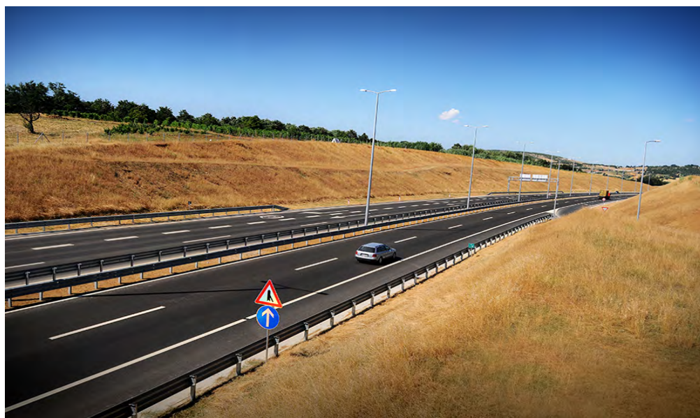
Existing motorway on Route 7 in Kosovo.
