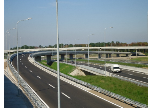
View of Banja Luka – Gradiška motorway (Mahovljani Interchange), operational since 2011. © JP Autoputevi Republike Srpske
