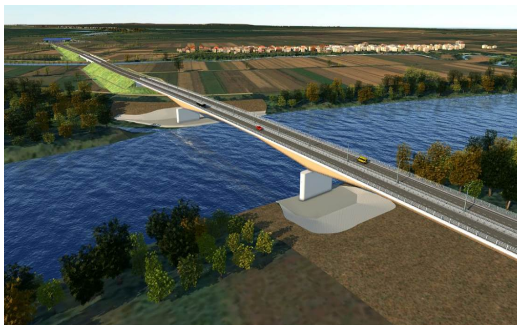
Proposed design for the cross-border bridge over the River Sava at Gradiška. © Ministry of Communications and Transport of Bosnia and Herzegovina
