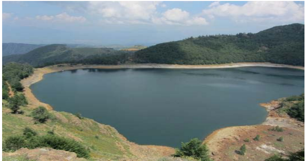
Ternoves Hydropower Plant, Albania
