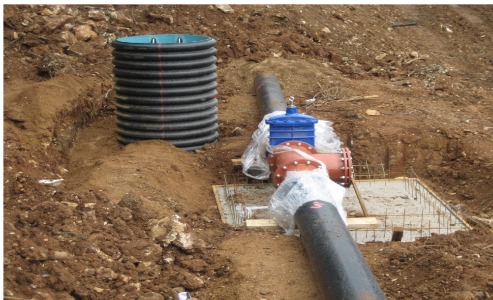
Construction of wastewater collectors, Bosnia and Herzegovina.
