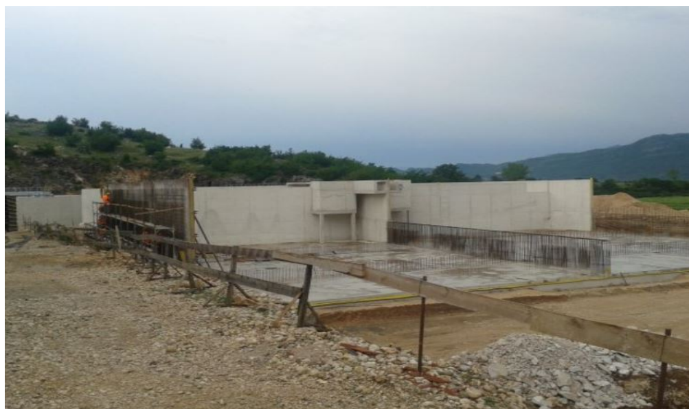
Wastewater treatment plant works, Montenegro.
