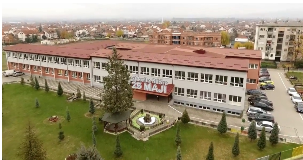
Primary school "25 May", Skopje (after rehabilitation works).
