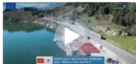
Rail R4 Bar-Vrbnica, Montenegro
