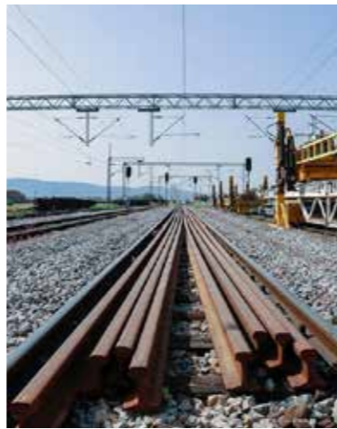
Albania on track for faster, safer railway March 2024
