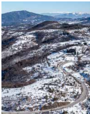
Road between North Macedonia and the Bulgarian border opens for traffic January 2024
